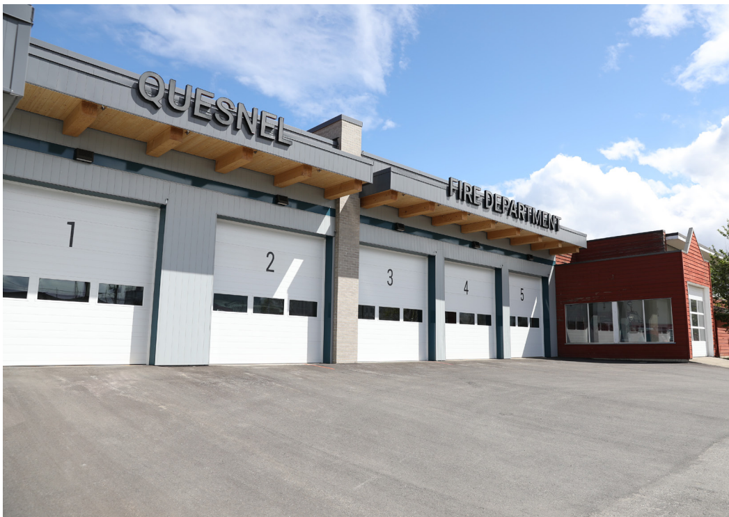
Quesnel's downtown Fire Hall renovation
