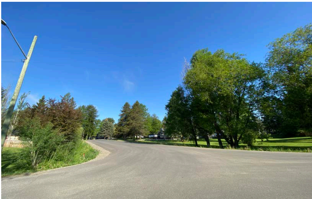
Lignin-modified asphalt pavement in South Quesnel
